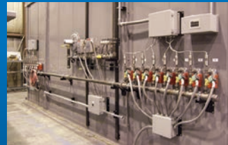
Pressure Transducer Monitoring Lines and Data Acquisition Control System
